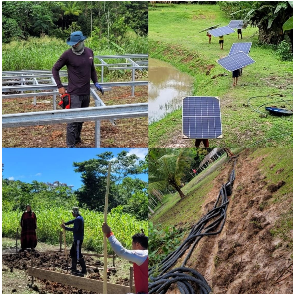
Figure 2: Efforts to transport and install solar energy systems.
